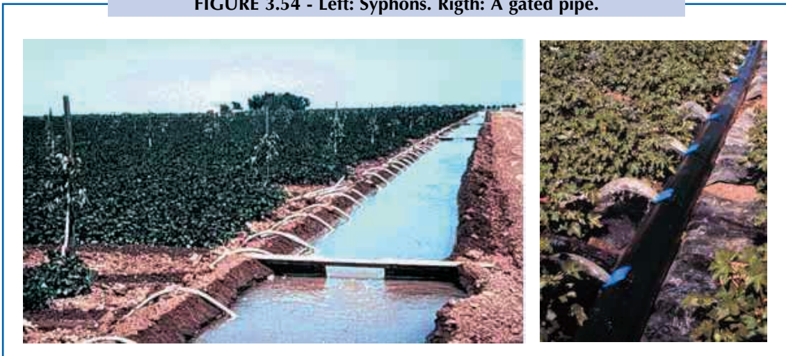
FIGURE 3.54 - Left: Syphons. Right: A gated pipe.
