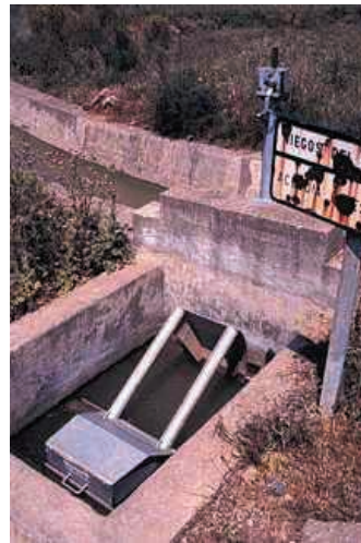
FIGURE 3.51 - Left: a gate for a farm turnout. Right: a Neyrpic gate.
