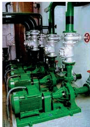
FIGURE 3.46 - Left: a rotodynamic pump powered by a tractor. Right: a pumping unit with rotodynamic pumps in parallel.
