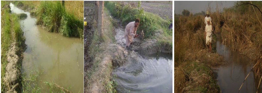
Figure-10: Unimproved Watercourses
