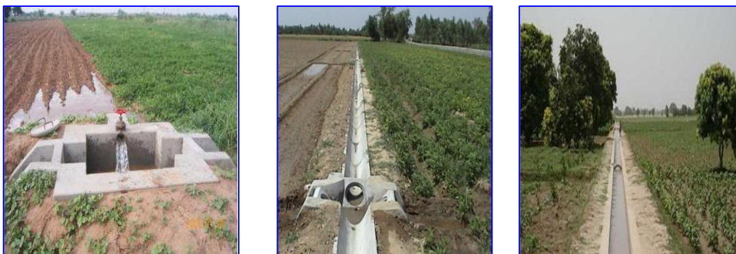
Figure-8: Glimpses of Lined Watercourse using Pipe, PCPS and Brick Lining
